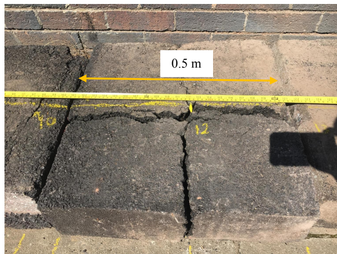
Figure 2: One of the tested asphalt slabs
