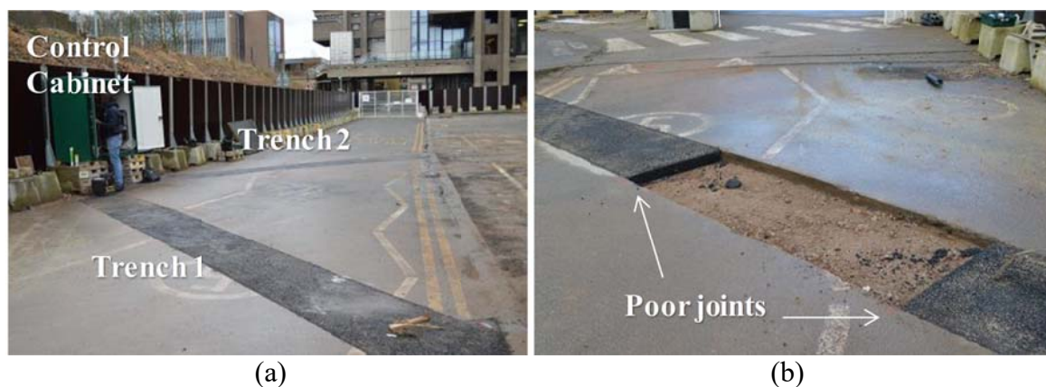
Figure 2: (a) The two reinstated trenches and (b) construction of the poor joints
