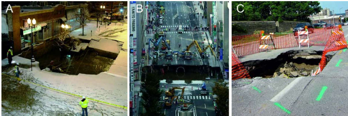
Figure 2 – Urban sinkholes attributed to soil piping resulting from broken or leaking water pipes removing material with subsequent collapse of asphalt capping layer. A) collapse at corner of Montrose Avenue and Honore Street, Chicago, caused by broken water transfer pipe (TheeErin on Flickr under a cc-by-2.0 licence), B) Large sinkhole in Fukuoka, Japan in November 2016 (Muyo on wikimedia commons under a cc-by-sa 4.0 license), C) Sinkhole in St Mary's Avenue, Omaha, attributed to leaking pipe (Courtney "Coco" Mault on Flickr under a cc-by-2.0 license).
