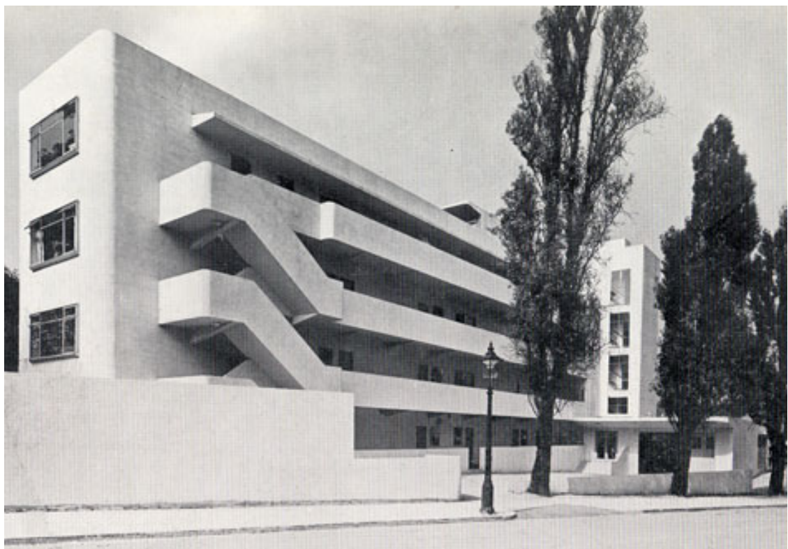
Figure 1: Lawn Road Flats, architect Wells Coates
