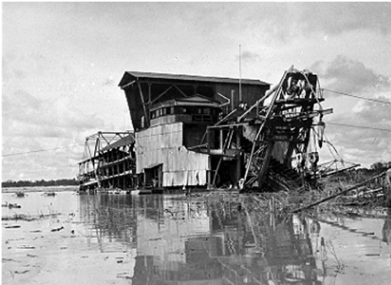
Figure 4: Tin bucket dredge north of Manggar, East Belitung, 1937. Credit: Tropenmuseum, Amsterdam.
