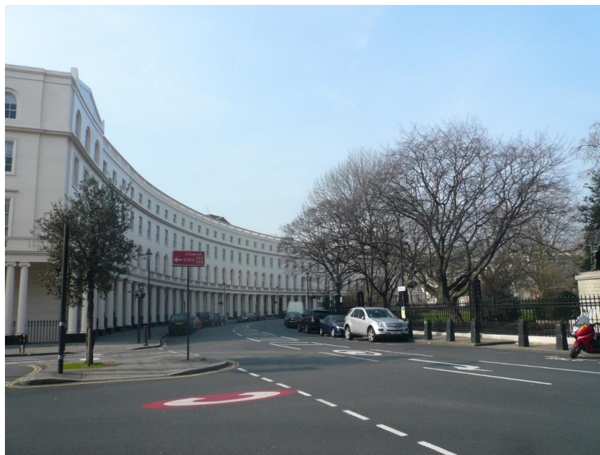
Figure 5. Park Crescent, London: redevelopment of post-war replica. The visually identical but more original part of the crescent is behind the photographer (photograph by P.J. Larkham, 2019).
