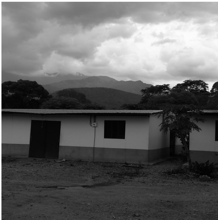
FIGURE 8.2 The asbestos houses in the FARC reincorporation zone. Photograph by the author.
