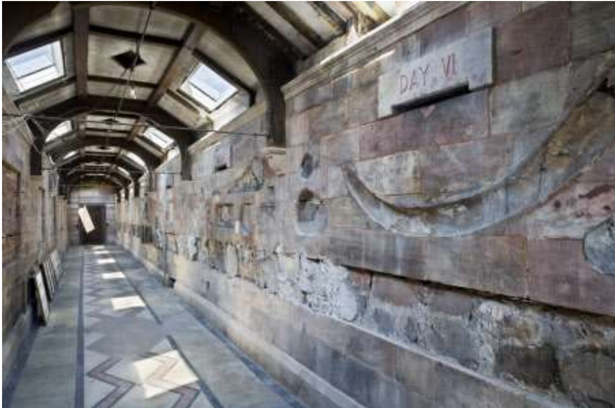
Figure 1. Biddulph Grange's Geological Gallery at an early point in the restorations - note the shaped impressions where fossils (now casts) fit literally into the walls, becoming part of the building. The long horizontal line is for sequential rock strata, and the sections above divide the gallery into Biblical days of creation - Day VI, in the foreground, has space for a mammoth tusk. (Image: National Trust)
