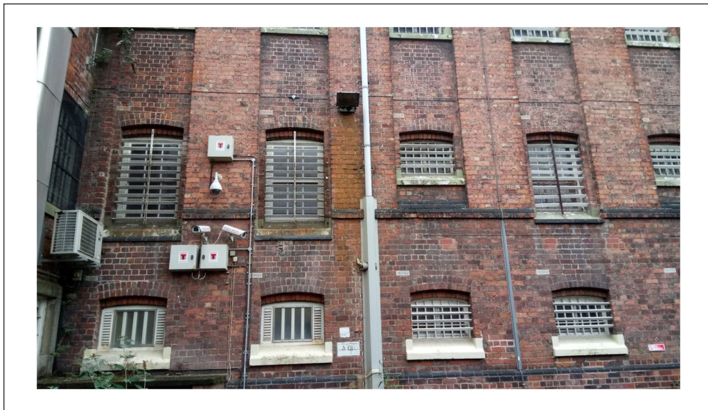
Figure 1. Exterior View of HMP Shrewsbury Showing Different Window Sizes, Security Cameras, and Pipework (Image Credit: Dominique Moran).
