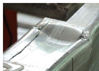
(b) Brittle cracking (STB80-A)
