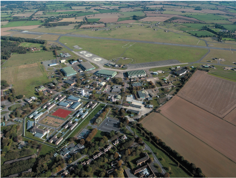
Figure 1. Aerial photograph of HMP Bure, formerly RAF Coltishall. The prison comprises the cluster of original military buildings (including H blocks) at bottom left, enclosed within a new perimeter wall, and centred around the original parade ground (now a sports field). Military aircraft hangars and the airfield itself are clearly visible, beyond the prison complex, at the top and centre. Source: John Fielding (CC BY 2.0)
